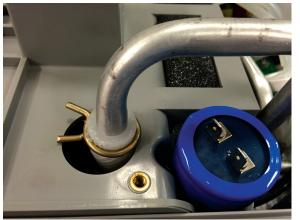
5. Remove the four (4) screws from the compressor cover using a Phillips screwdriver.
